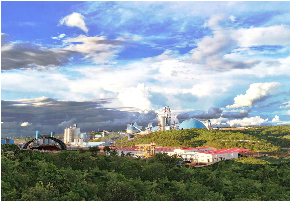
An aerial view of the newly opened US$ 500 million Investment Sinoma Cement Plant in Chongwe District
