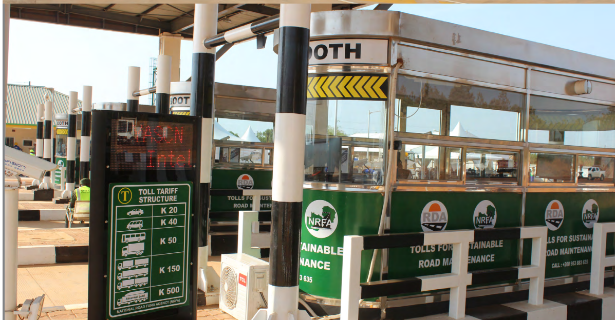
Michael Chilufya Sata Toll Plaza along Ndola-Kitwe Road
