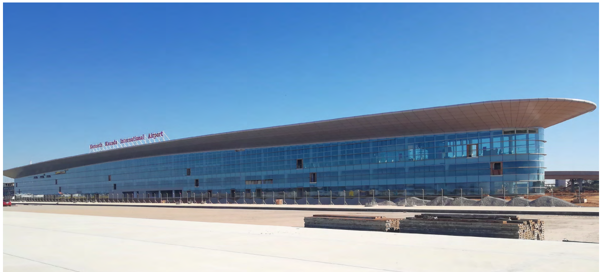
Newly constructed Kenneth Kaunda International Airport in Lusaka
